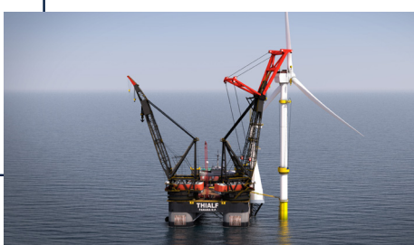
FULL WTG LIFT FROM DECK TO FOUNDATION | 5
