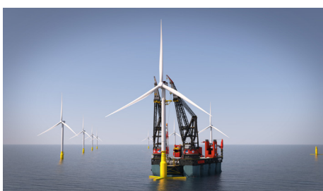
DUAL CRANE FULL WTG LIFT TO FOUNDATION
