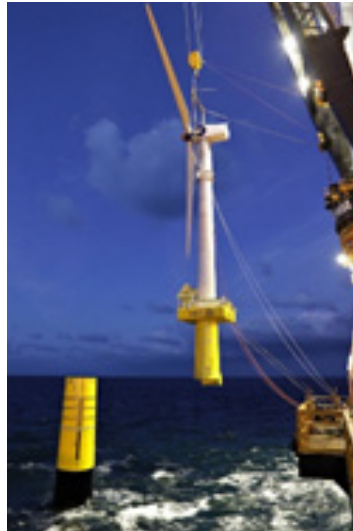
WTG INSTALLATION DURING SJOR DEMONSTRATION PROJECT
